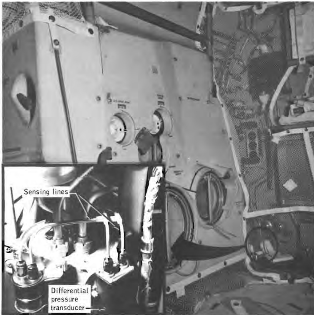
Figure 14-25.- Glycol pump sensing lines.
