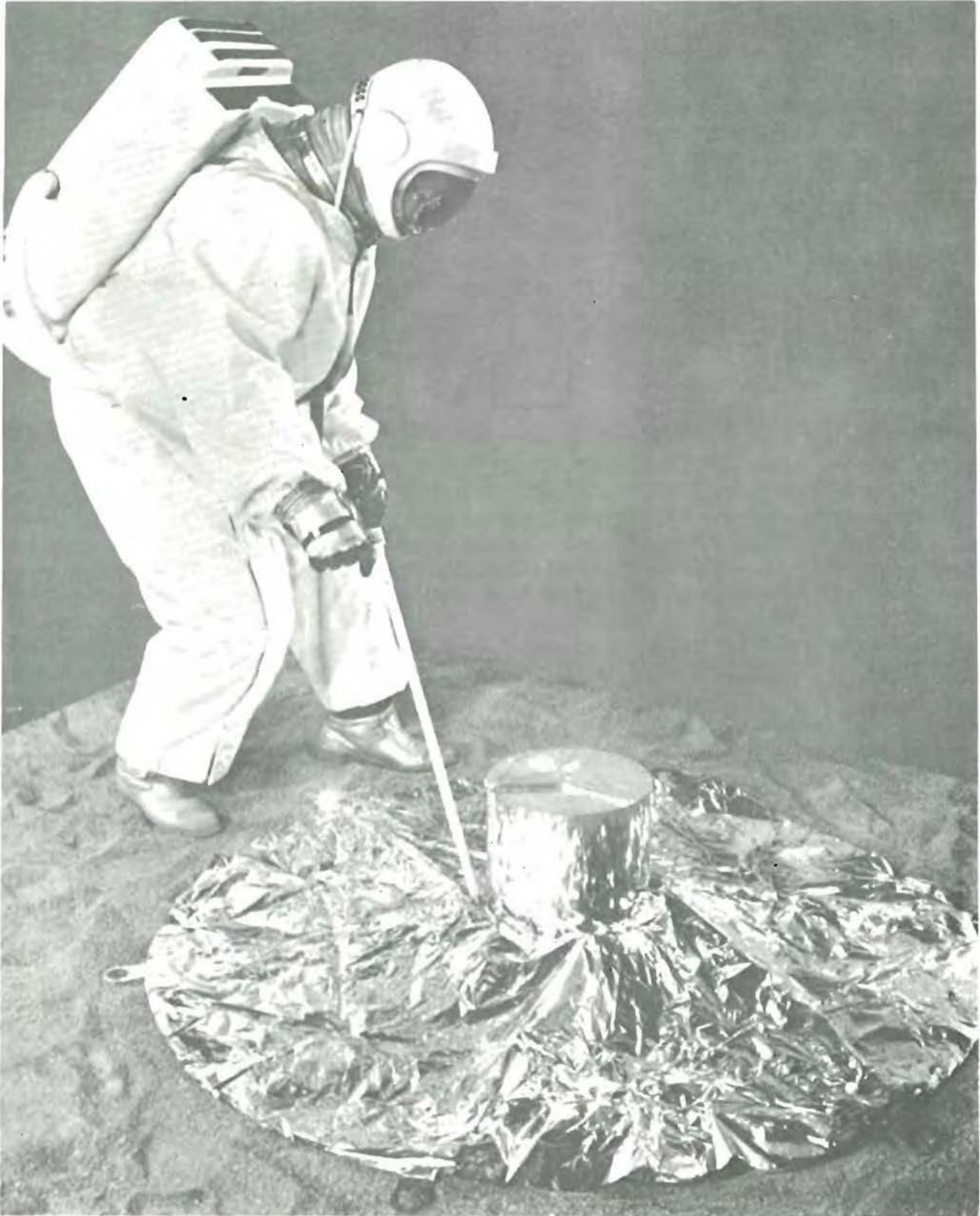
Figure 4-5. PSE Shroud Deployment and Experiment Leveling
