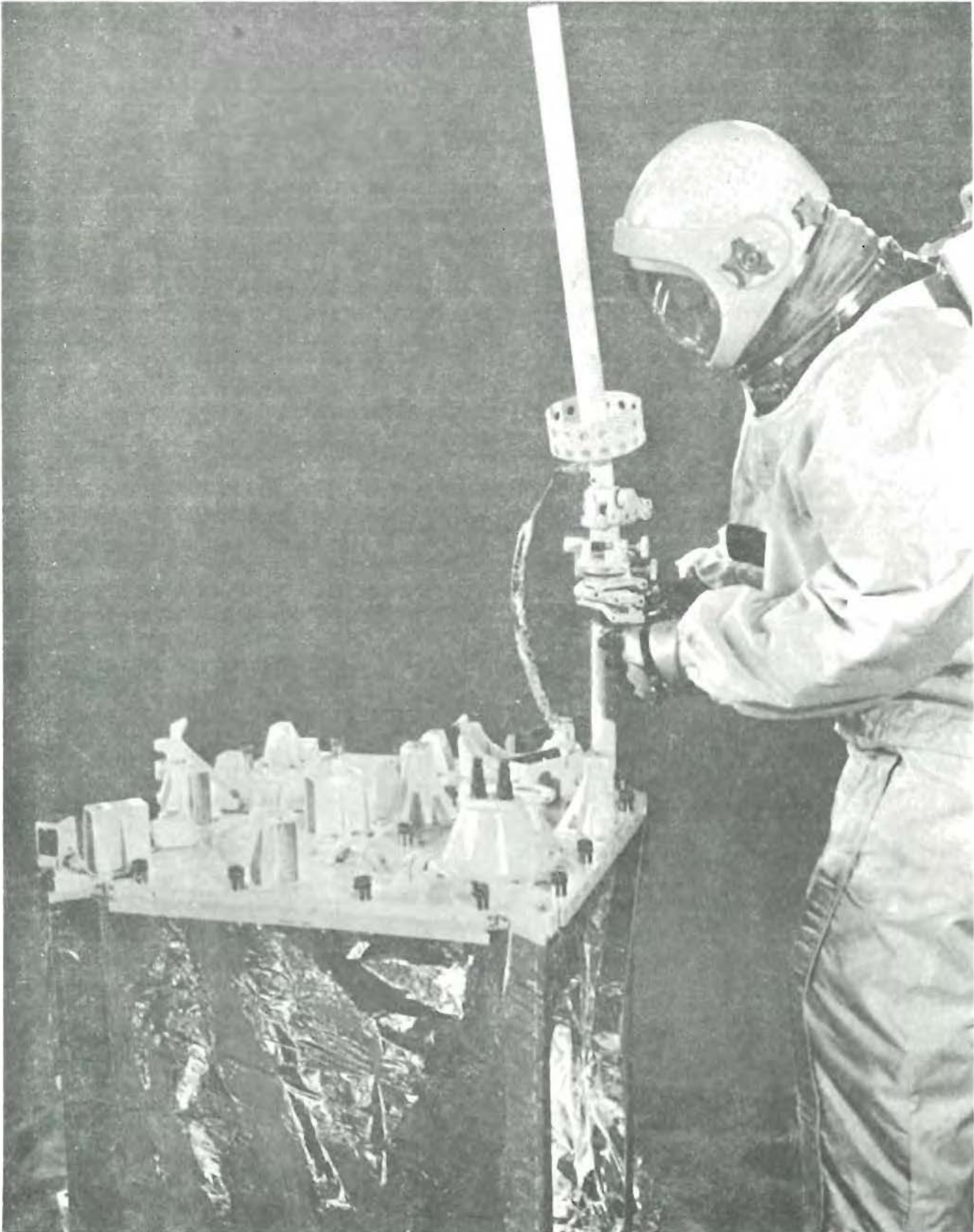
Figure 4-7. Antenna Aiming Mechanism Alignment
